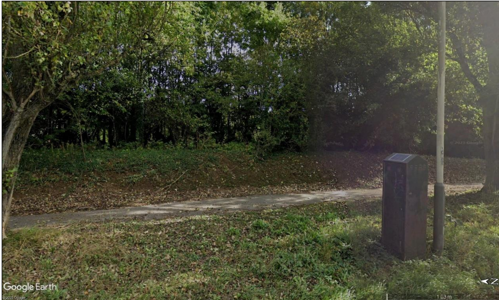
View towards reflecting panels from road receptor 31 (representative of the extent of screening for road section 31-33)
