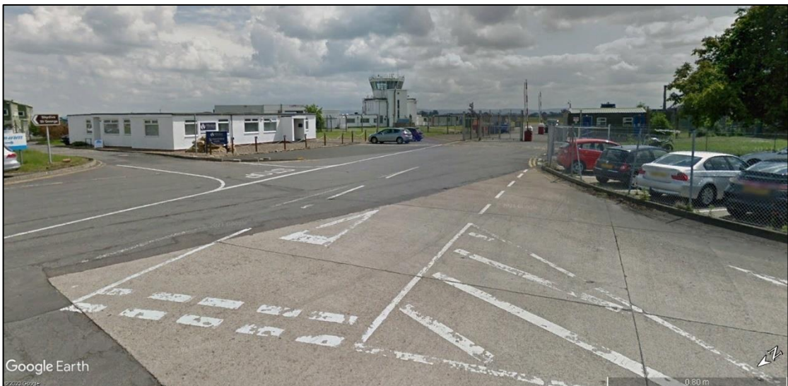
Figure 59 ATC Tower at Teesside International Airport – street view image
